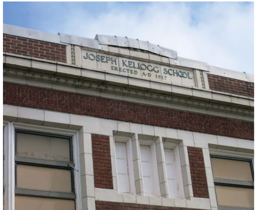
Existing Main Building Parapet Coping and Windows
