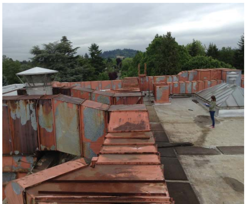
Existing Roof and Rooftop Mechanical System
