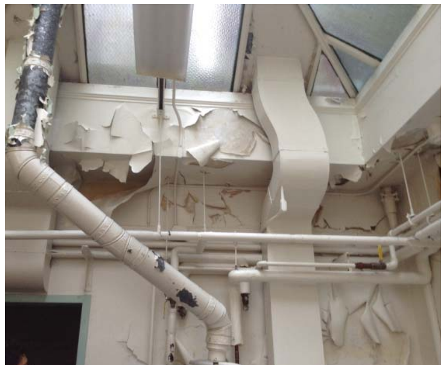
Existing Skylight and Building Systems
